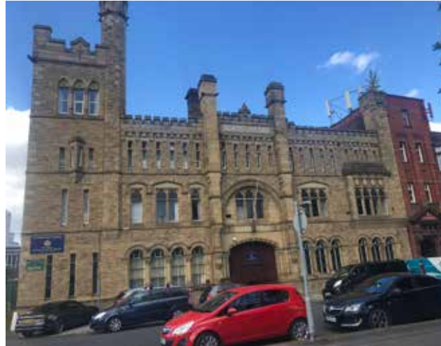
1. DRILL HALL, ARDWICK GREEN NORTH, GRADE II (List No. 1207590)
