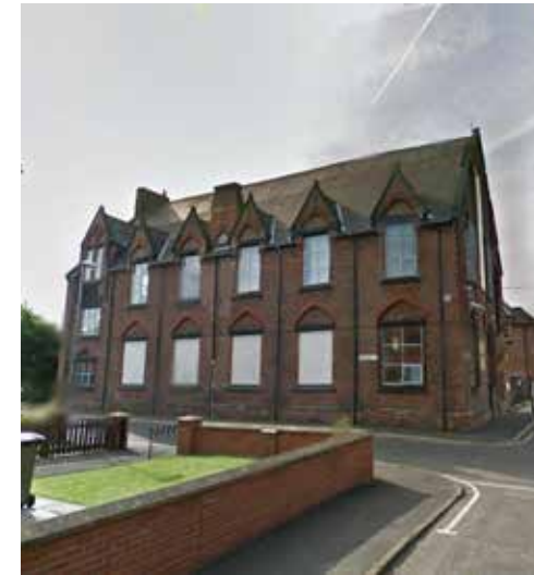
3. The Old School House, Thirsk Street
