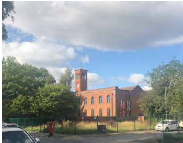
8. FORMER CHURCH OF ST THOMAS, ARDWICK GREEN NORTH, GRADE II (List No. 1197828)
