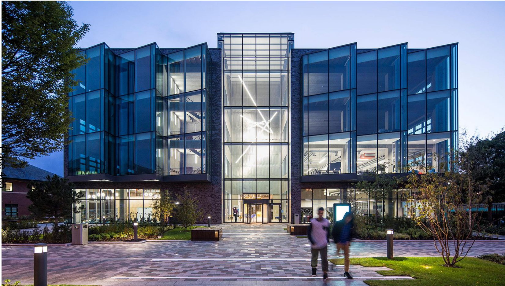
Figure F: Precedent Image for Commercial Research Building – Bright Building, Manchester Science Park (Source: BDP)
