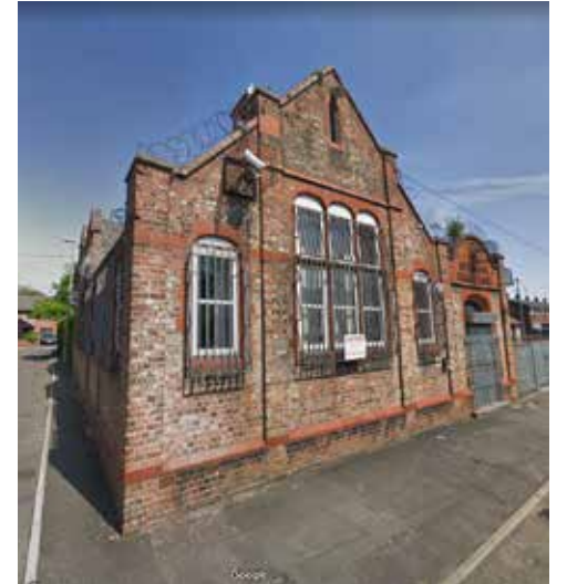
4. The Old School House, Thirsk Street
